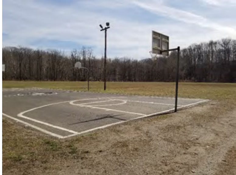
Photo 22: Existing basketball court
