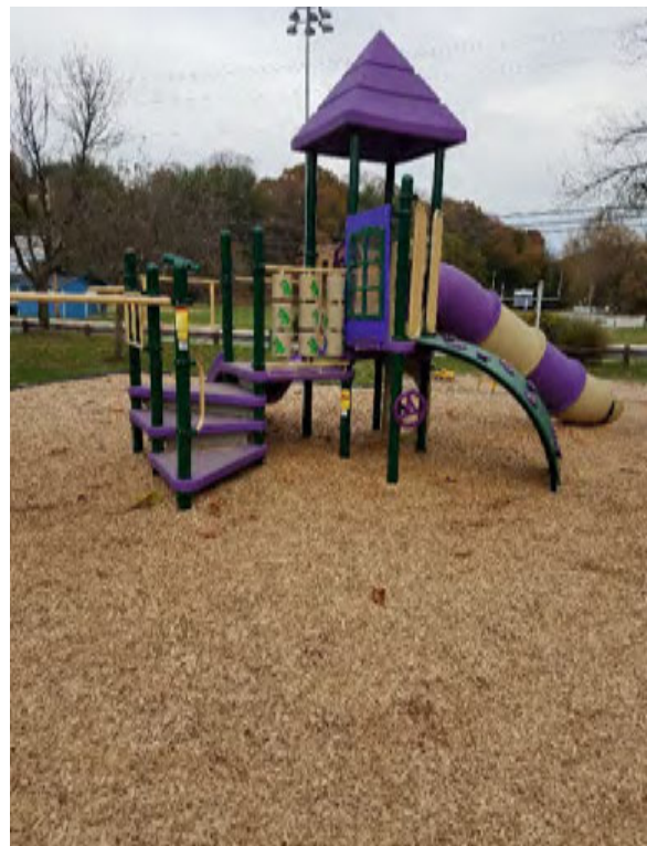
Photo 25: New play structure
