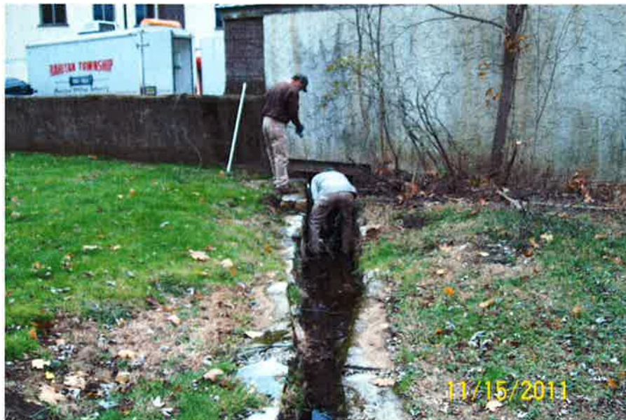
Photo No. 5 – Positioning the camera in the stone masonry channel.
