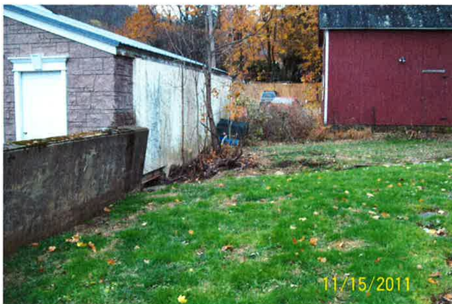
Photo No. 4 – Upstream access point at stone masonry channel.
