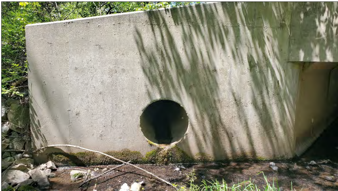
Photo 8: Typical 2-foot diameter cement stormwater pipe observed in both reaches.
